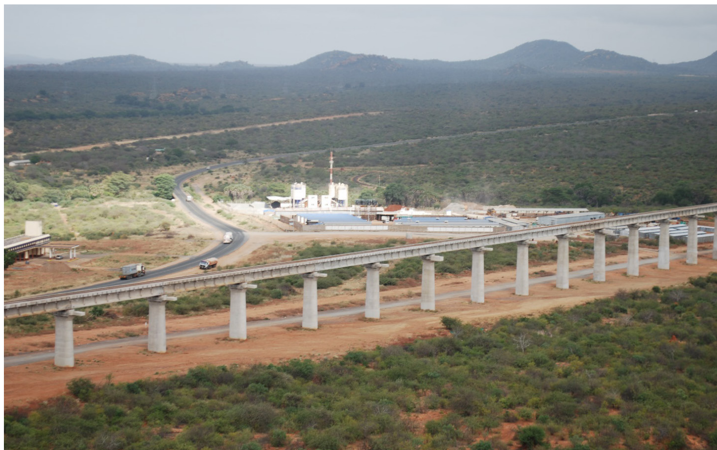
Plate 7.11: Aerial view of the SGR Tsavo River super-bridge, with underpass for use by wildlife. Next to it is the Mombasa-Nairobi highway. An overpass allowing animals to cross the highway needs to be urgently considered. Photo: courtesy Richard Moller/Tsavo Trust.
